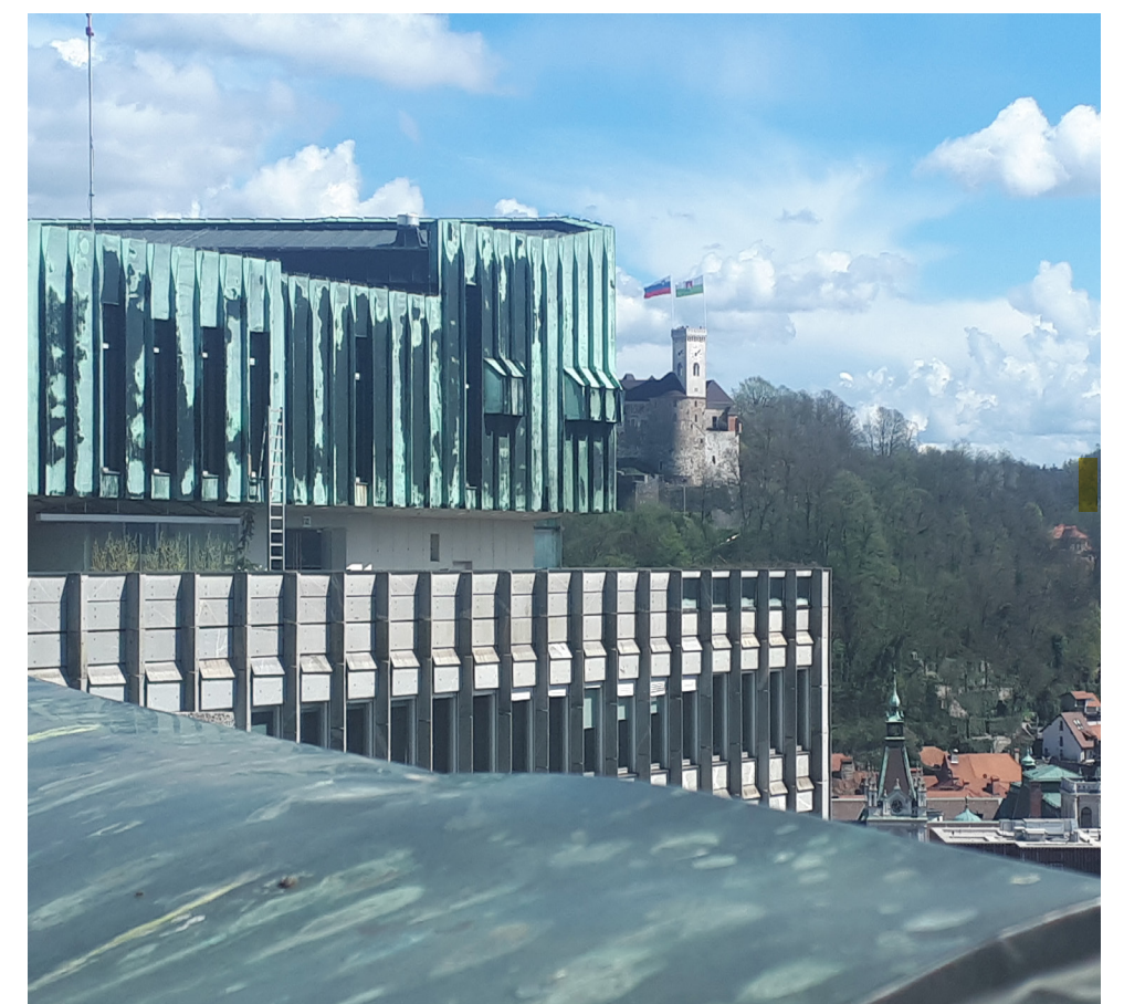
Edvard Ravnikar: Republic Square towers, 1976.
